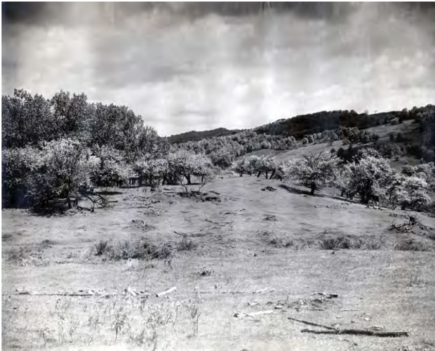
Fig. 1. Photograph taken in 1905 showing the remains of the foundation of the Joseph Smith Sr. home where Joseph Smith Jr. was born December 23, 1805. Photograph courtesy Church History Library.
