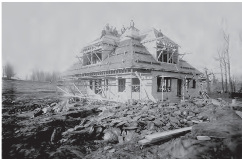
Fig. 3. The Memorial Cottage under construction, 1905. Photograph courtesy Church History Library.
