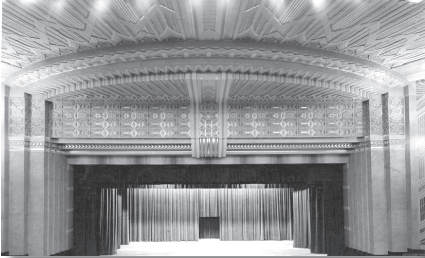
Early view of the Ogden High School auditorium, date unknown. Photograph courtesy Stewart Library Special Collections, Weber State University.
