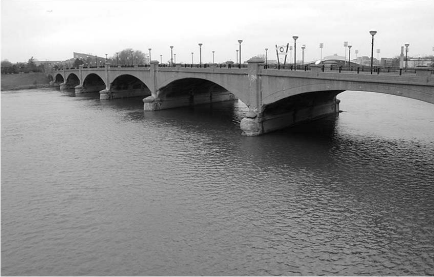
Image 8. Bridge over the White River, Indianapolis, Indianapolis, County, Indiana.
