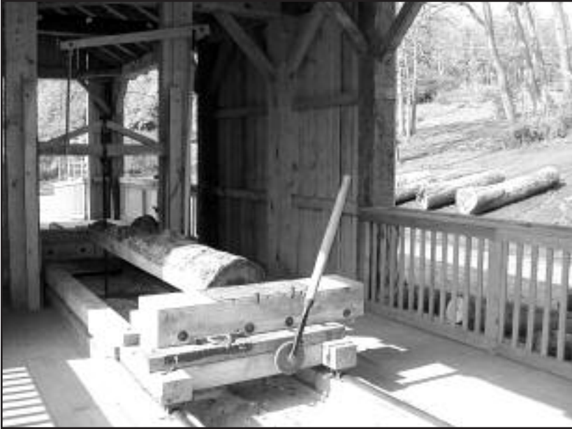
Portion of the reconstructed sawmill located in Kirtland Flats, 17 May 2003. Photograph by Alexander L. Baugh.
