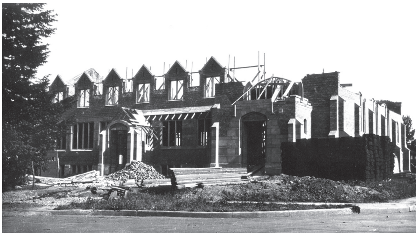
The Moscow LDS Institute of Religion under construction, summer 1928. Photograph courtesy Moscow LDS Institute of Religion, Moscow, Idaho.
