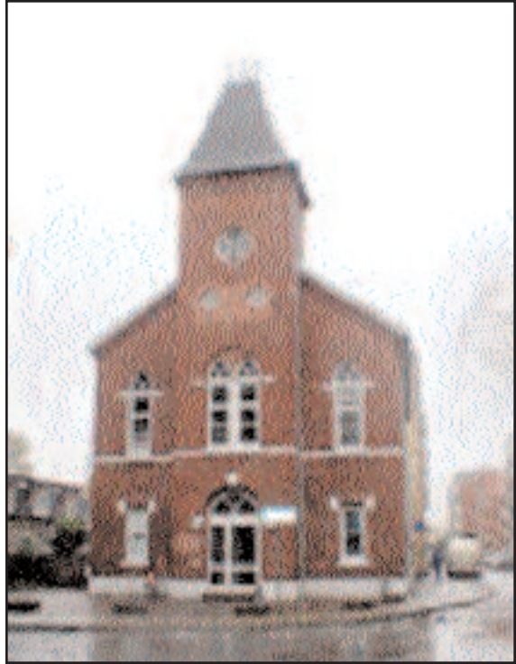
Aalborg LDS Chapel, Denmark Photo by Alexander L. Baugh
