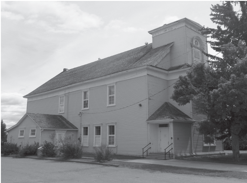
Former LDS meetinghouse in Raymond, Alberta, Canada, May 2012. The building was used as an LDS meetinghouse from 1912–1929. Photograph by Gary L. Boatright.
