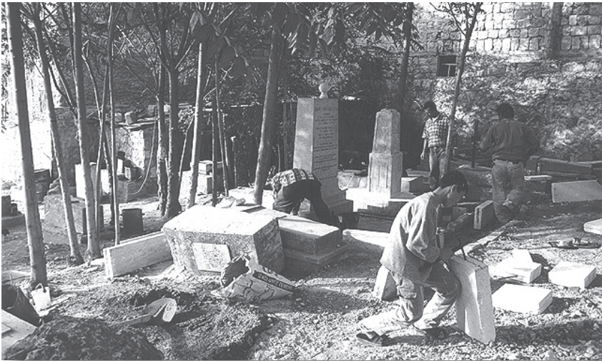
Stone masons and landscape engineers preparing the foundation for a wrought iron fence to surround the gravesites of Joseph W. Booth and Emil J. Huber, 2000. Photograph by James A. Toronto.
