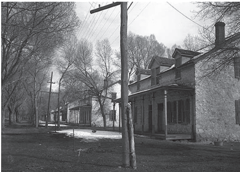
Several buildings at Fort Cameron which later served as dormitories for students who boarded at Murdock Academy. Photograph courtesy Church History Library, Salt Lake City, Utah.
