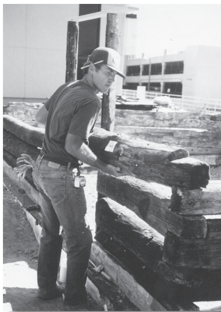
Don Enders erecting Deuel log home, Salt Lake City, Utah, 1985. Don's first project as lead was moving and restoring the 1847 log home of the Deuel family, situated between the LDS Family History Library and the LDS Church History Museum in Salt Lake City. Photograph courtesy Donald L. Enders.
