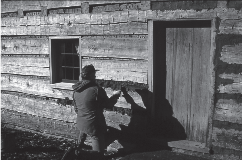
Donald L. Enders chinking the exterior logs of the restored Joseph Smith Sr. log home, Palmyra, New York, 1998. Photograph courtesy Donald L. Enders.
