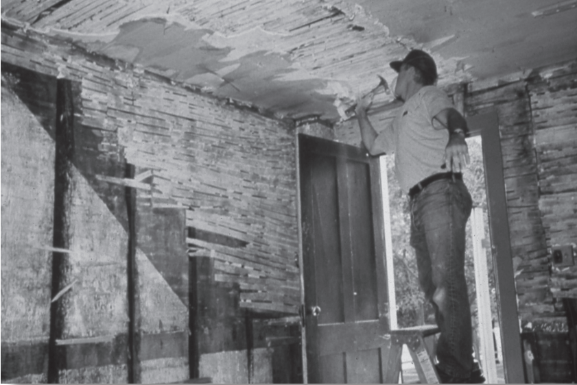
Donald L. Enders removing surface materials in the Joseph Smith Sr. frame home, Manchester, New York, 2000. Photograph courtesy Donald L. Enders.
