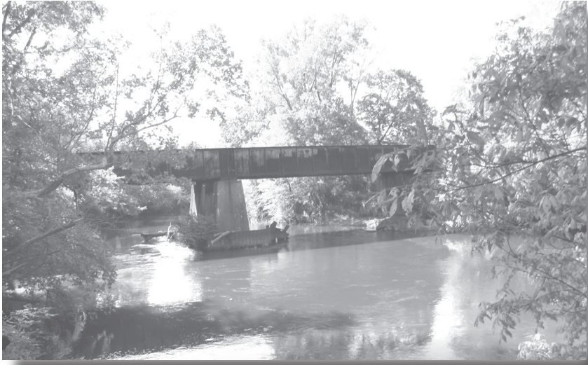
Fig. 7. Nottoway River railroad bridge, May 9, 2013, location of the Battle of the White Bridge on May 8, 1864. Photograph by Cindy B. Hoffman.
