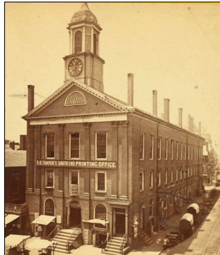
Boylston Market, Boston. Boylston Hall was located on the building’s third floor. Photograph by John B. Heywood, ca. 1860-1870. digitalgallery.nypl.org .
