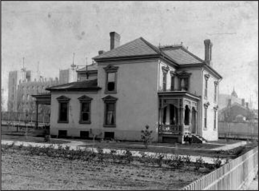
Home of William B. and Harriet Ann Preston on 74 West North Temple, Salt Lake City, Utah. Salt Lake Temple is under construction in the background. Picture taken ca 1887. William was presiding Bishop of the LDS Church from 1884 until his death in 1908.
