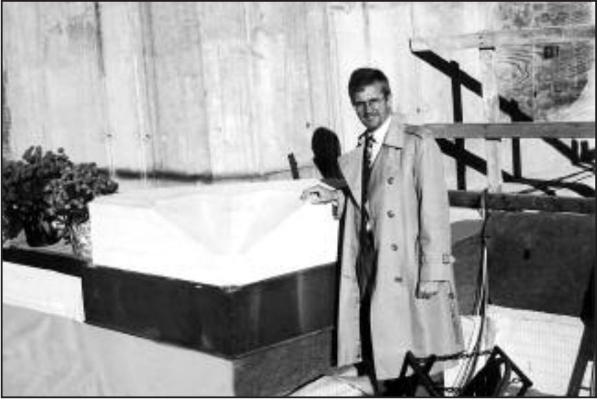
Roger Jackson at the southeast cornerstone, 5 November 2000. On this date, a cornerstone ceremony was conducted and presided over by LDS Church President Gordon B. Hinckley at each of the four corners of the building. Photograph courtesy of Roger P. Jackson.
